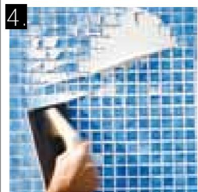
ezarri recommends the use of CG2 class grouting. Epoxy joints within the RG class should be used for places that require chemical sterilisation or high resistance to moisture.
